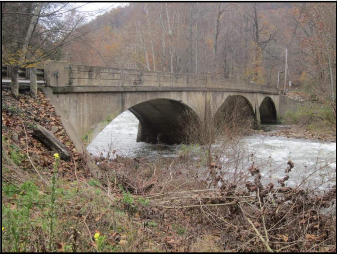
North Elevation. View SW (WVDOH 11-8-2018)
