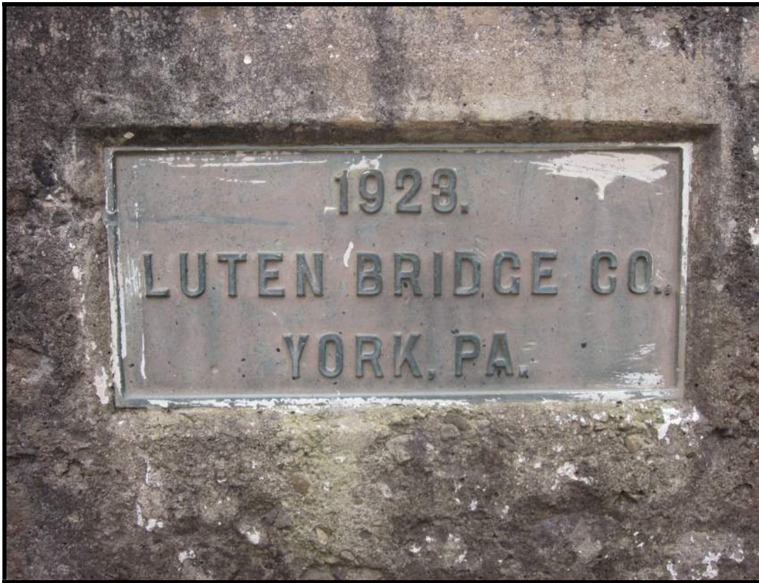
Plaque on North/Upstream Side Railing. View North (WVDOH 11-8-2018)
