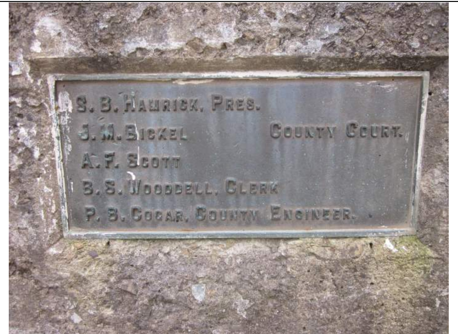
8. Plaque on South/Downstream Side Railing. View South.
