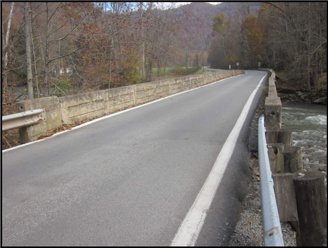
West Approach. View ENE (WVDOH 11-8-2018)
