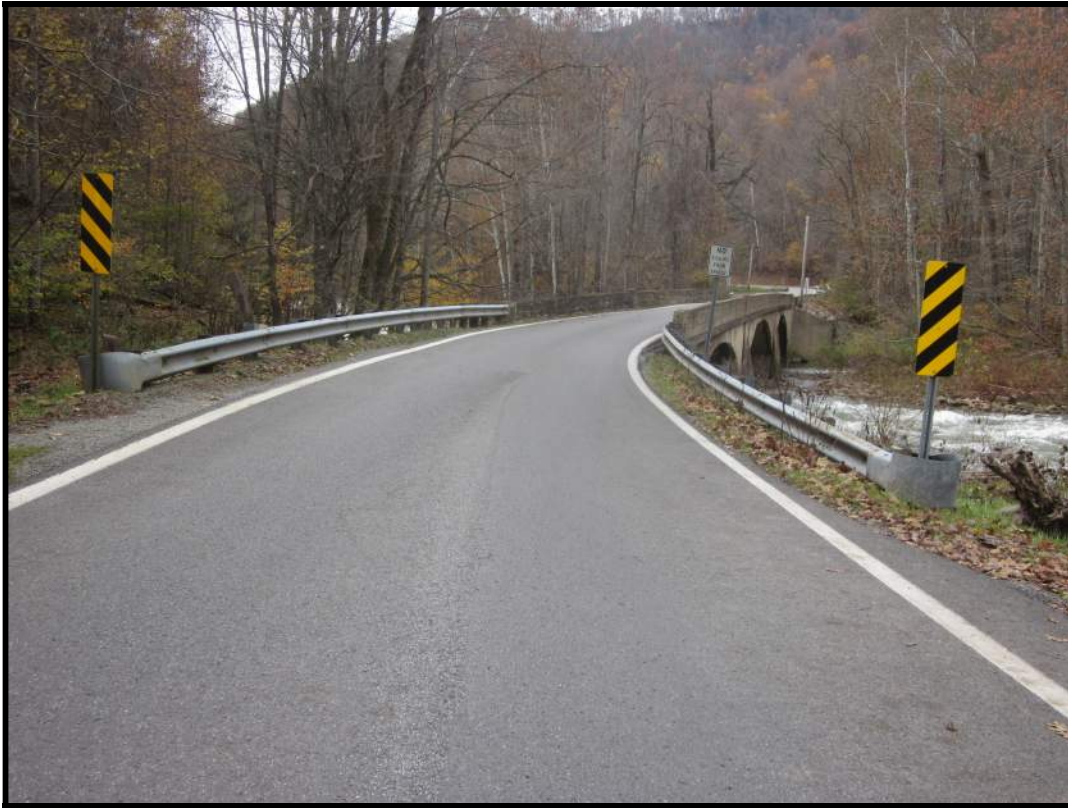
East Approach, with guardrails. View W (WVDOH 11-8-2028)
