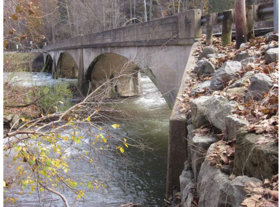
4. North Elevation. View Southeast.
