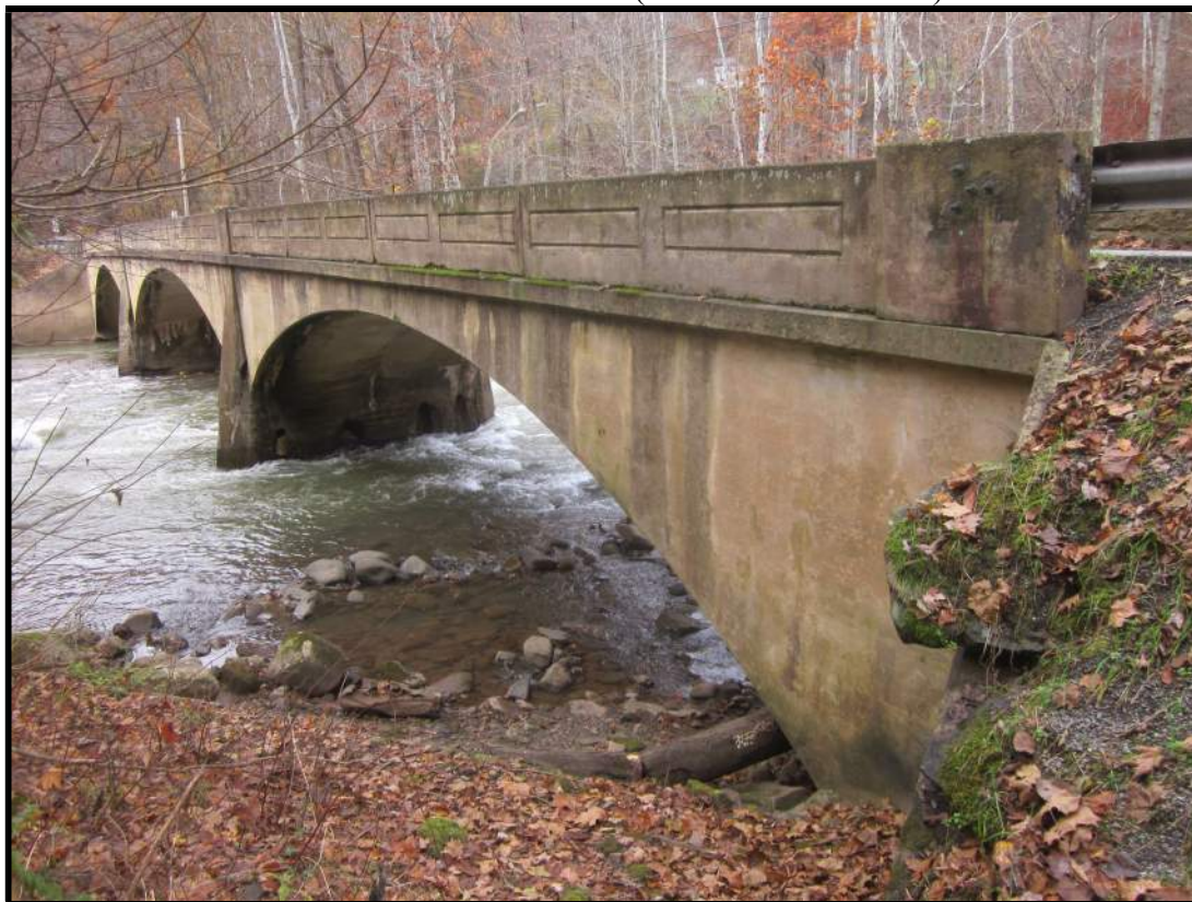
South Elevation. View NW (WVDOH 11-8-2018).
