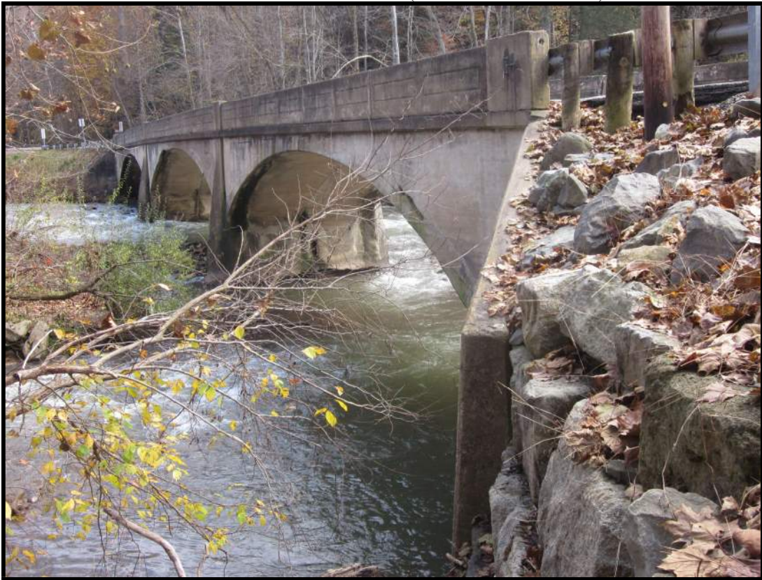
North Elevation. View SE (WVDOH 11-8-2018).
