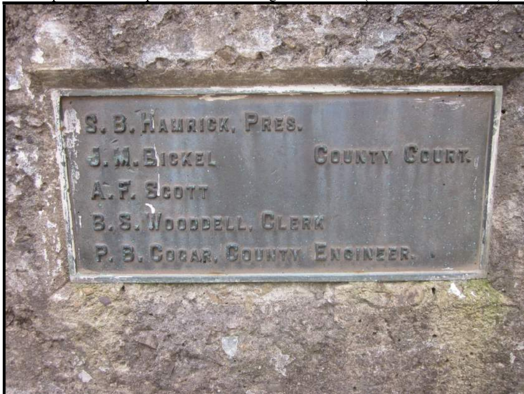
Plaque on South/Downstream Side Railing. View South (WVDOH 11-8-2018).
