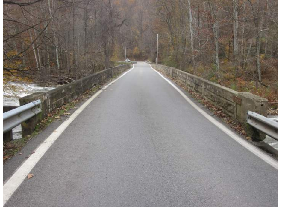
6. East Approach. View West/Northwest.
