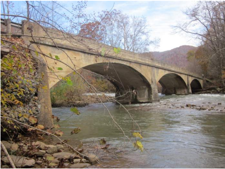
1. South Elevation. View Northeast.
