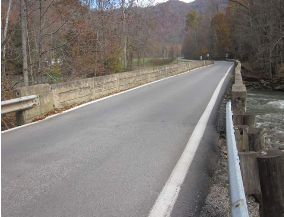
5. West Approach. View East Northeast.
