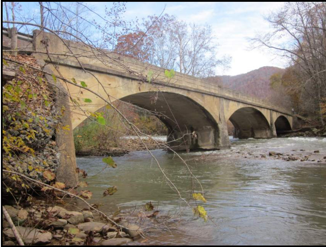
South Elevation. View NE (WVDOH 11-8-2018).
