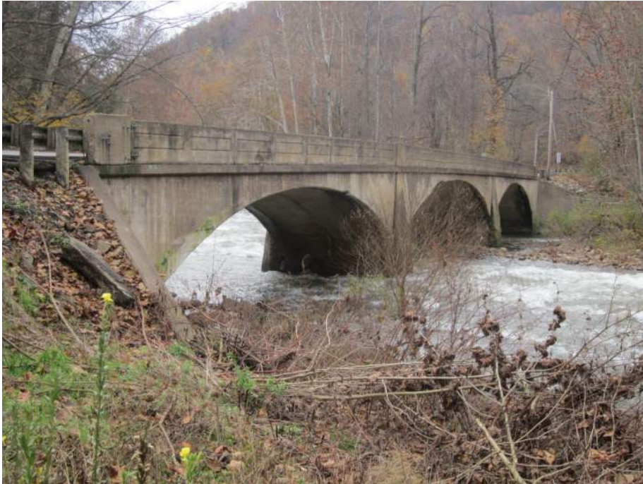
3. North Elevation. View Southwest.
