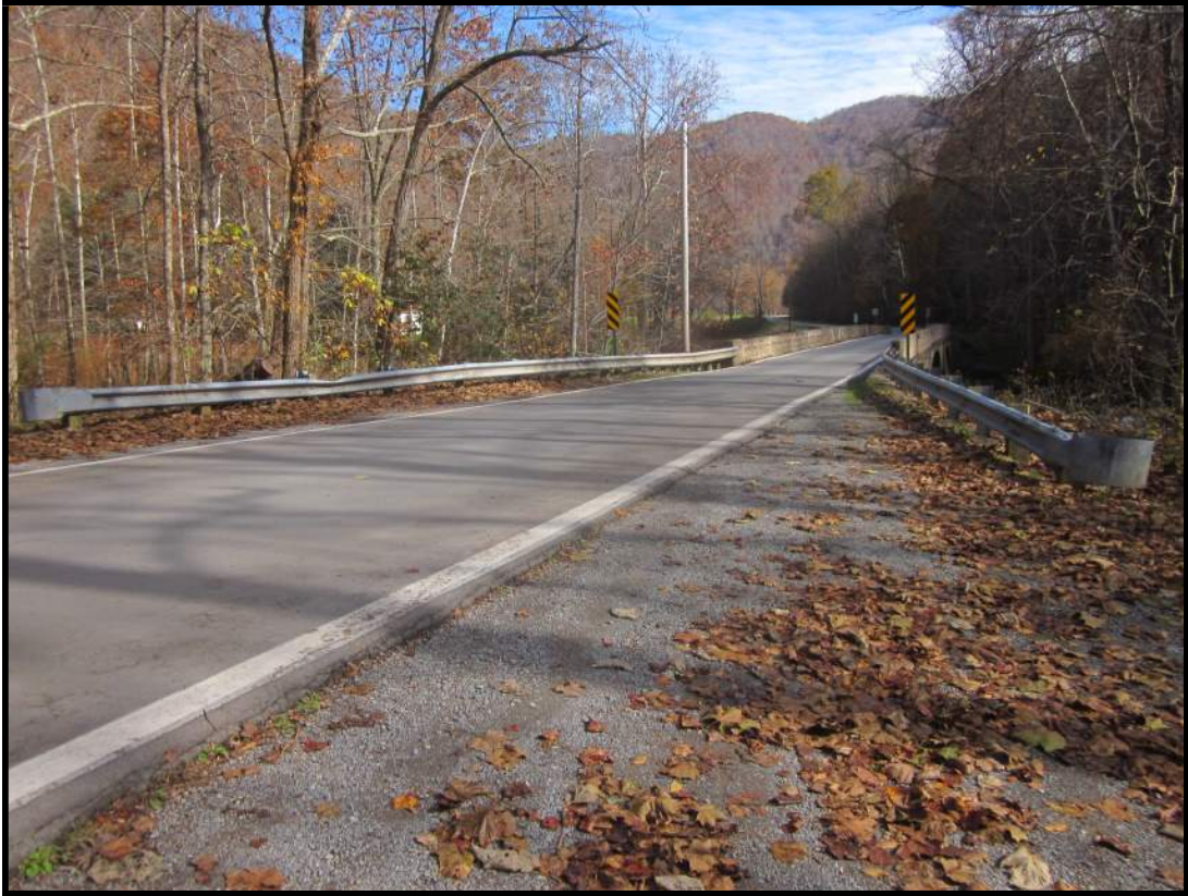
West Approach, with approach guardrails. View E/NE (WVDOH 11-8-2018).
